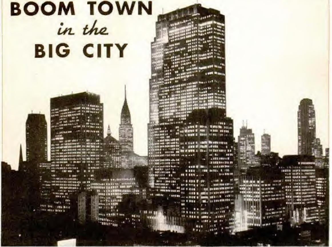
This was Boom Town—New York's Rockefeller Center—before the dim-out. Now all's dark above 15th floor
